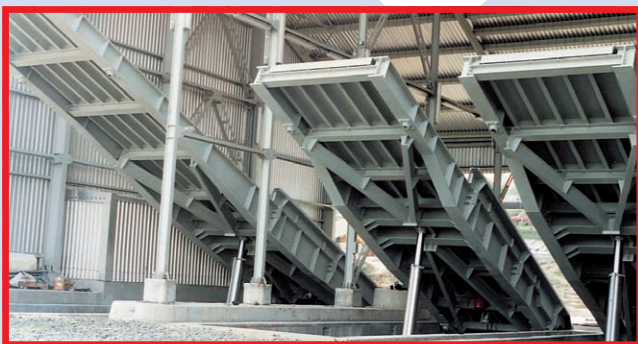
Truck dumper station
